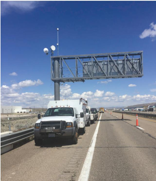
*NDOT installing Redline's Virtual Fiber™ radios on a DMS along I-80*
